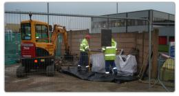
Excavation can generate spoil on occasion, in this instance spoil is required to be placed in dumpy bags for removal and storage. This requires the use of a metal frame to keep operatives away from the loading operation. These pictures show the operatives acting as spotters from outside the segregation zone and only entering the segregation zone to change the bags once the thumbs up has been received and the plant is isolated.
