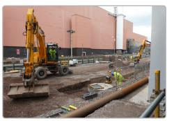
Operatives are required to enter the plant/ vehicle zone to complete a task e.g. pouring concrete from skip, installing or removing trench boxes, working in manhole.
