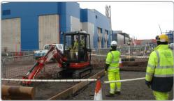
An operative is required to take a level from an excavation whilst the plant is in operation he remains outside the segregation zone. Only after the thumbs up and machine is isolated does he enter the segregation zone to take a level. These pictures demonstrate a controlled, methodical and sequenced approach to close proximity working, within a managed mobile segregation zone.
